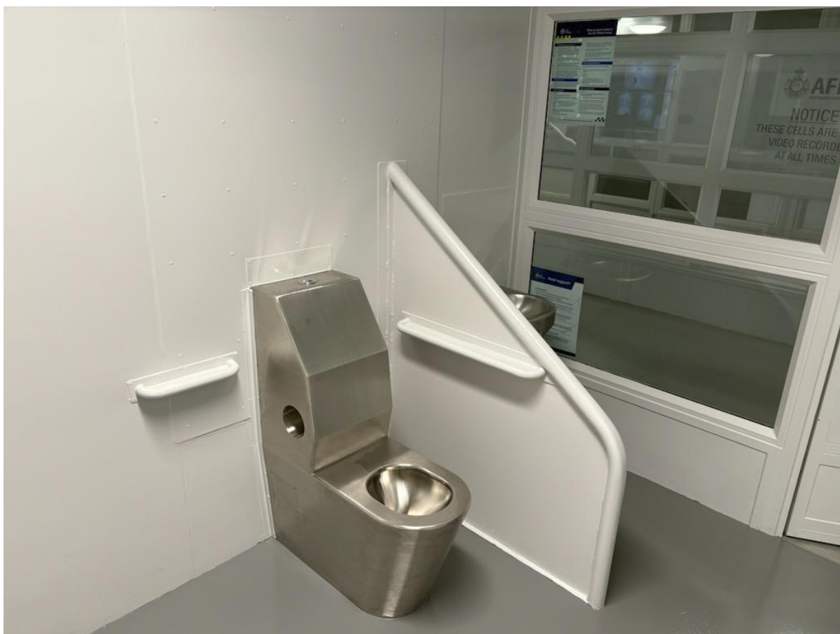
Photo: The new toilet including grab rail and privacy screening within the reasonable adjustment cell at the ACT Watch House (4 September)
